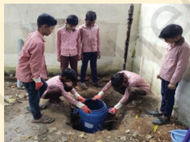
Figure 6.8: Students making a soakpit
